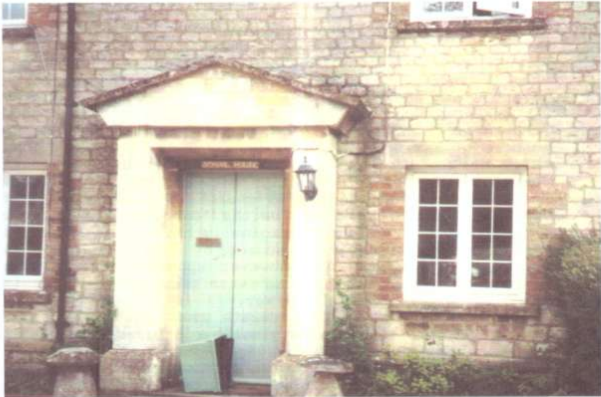
Fig.11. The Old School House at Bourton - a good example of Portlandian limestone of local origin. Note the well formed - dressed- and well coursed limestone 'bricks'.
