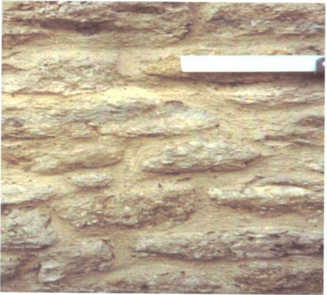
Fig.8 . Where not visible to the neighbours, house walls were built of virtually undressed rag stone and are often rich in fossil shells or pieces of fossil coral and are as much limestone as grit. The stones used in the construction of this side wall are roughly ellipsoid in shape which allows only a crude coursing. The white marker is about 15 cm long).
