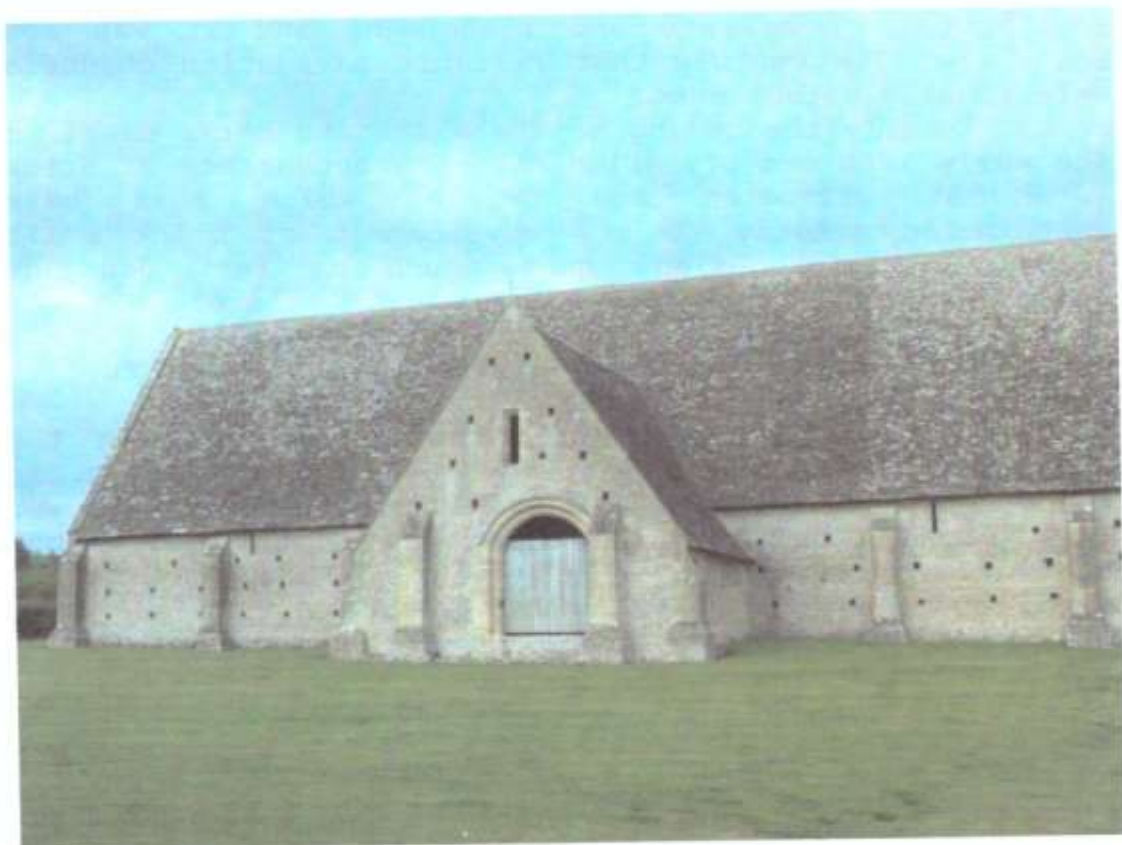
Fig.10 . The Great Barn at Coxwell The massive roof is tiled completely with Stonesfield slates.
